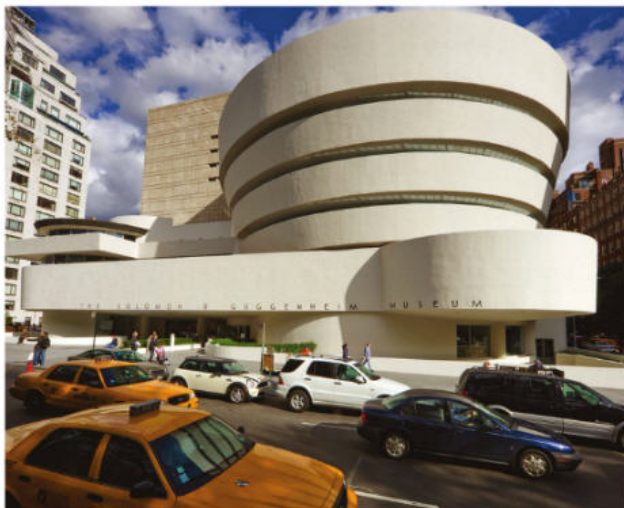
Quality-control measurements can play a key role in ensuring proper surface preparation, substrate moisture, environmental conditions, and coating thickness and adhesion. Restoration of the exterior of Frank Lloyd Wright's Solomon R. Guggenheim Museum, shown here, was a subject of a feature story in Journal of Architectural Coatings (now D+D ) in 2009. Photo by David Heald © The Solomon R. Guggenheim Foundation, New York
